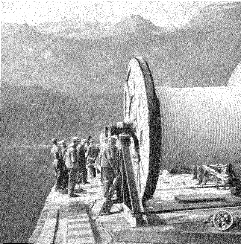
Reel of cable on a cable-laying lighter. The terrain at a typical deep fiord is shown here.
