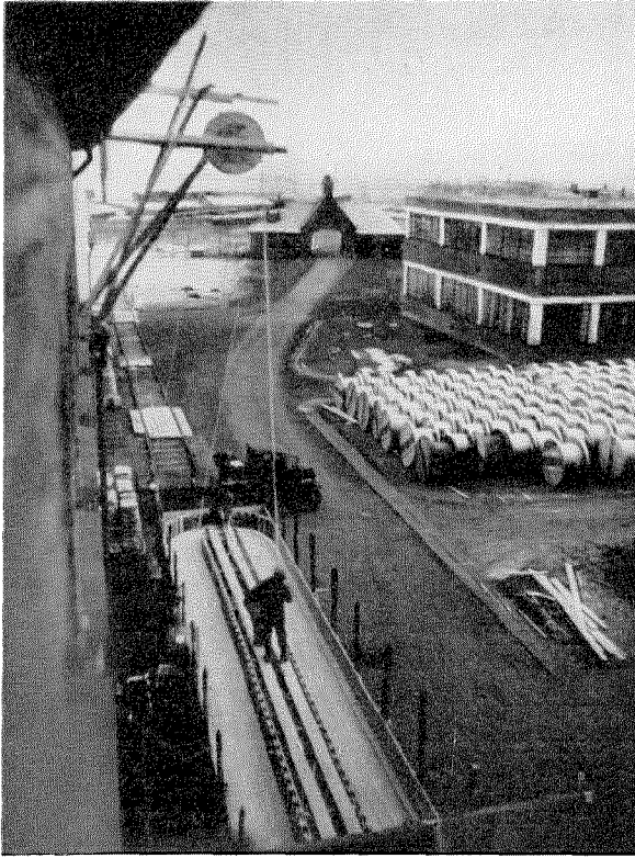
Cable being coiled on a railway flat car for transportation to the cable ship. Several such cars are necessary when a cable of considerable length is shipped.
